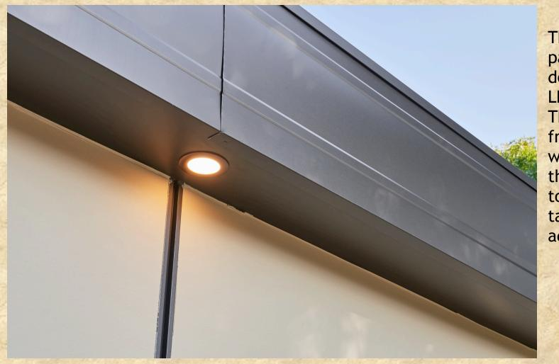
The dark parapet is dotted with LED lights. The framework was raised three inches to match the taller addition.
