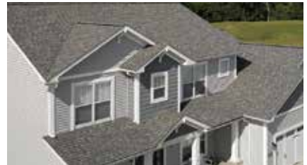
ROOFING AND VENTILATION
