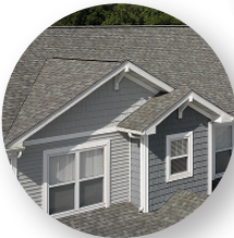
Roofing and Ventilation
